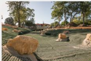
Brownhill Creek Pyramat and Stepping Boulders January 2019
