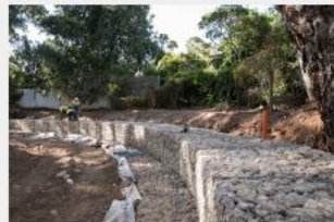
Brownhill Creek Upgrade JWS Morris Gabions January 2019
